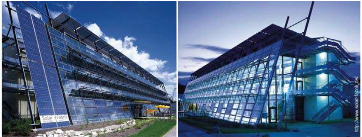
Fig 27: Inclined PV Integrated Façade of Solar-Fabrik Building, Freiburg, Germany ( http://www.solar-fabrik.de/ )
